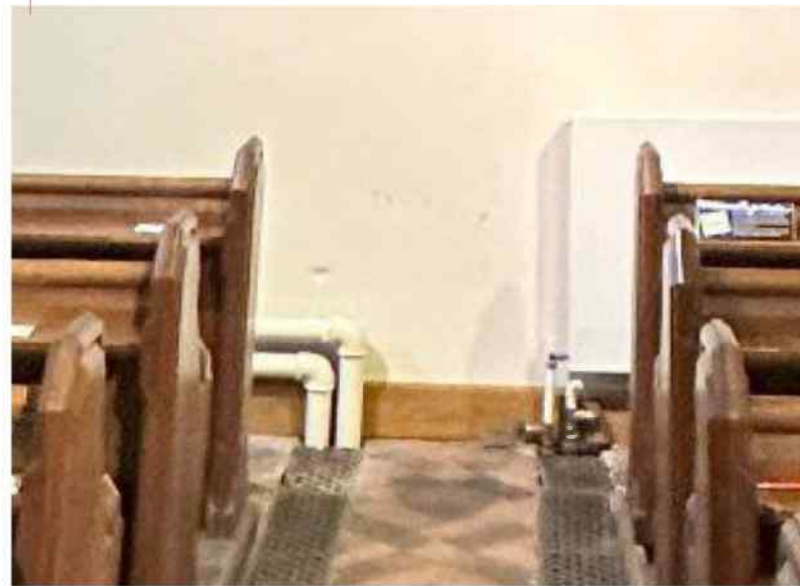
Existing supply pipework to be removed and capped
