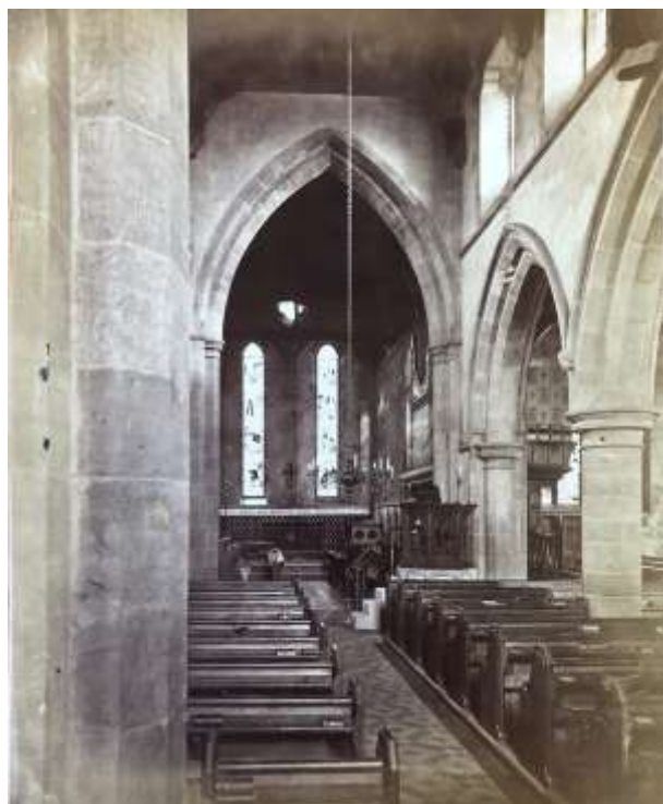
Chancel, nave and south aisle, c. late 1870s
